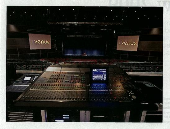
The Venue's audio system **Includes two Yamaha** PM5D-RH digital consoles; one Yamaha DME24N, one DME80-ES, and two **DME64N digital mixing** engine controllers; and a Meyer Sound line array. The video setup features three **Digital Projection International Lightning** 30isx+ projectors, screens by Draper and Lesna, and a Ross Vision QMD/X series digital switcher for video control.
